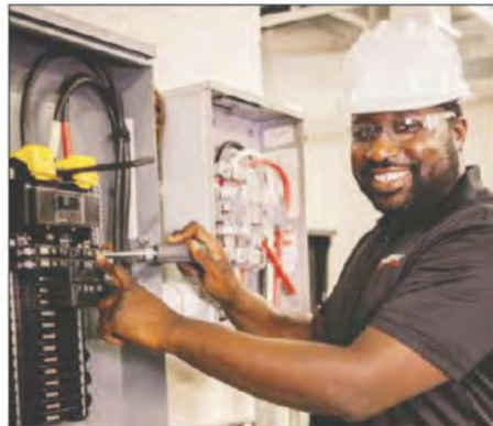
A CFK electrical apprentice checks an electrical panel in class on the Upper Keys Center.
