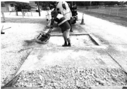
County road crews repair a section of road damaged by iguanas that tunneled next to an old culvert to lay eggs. MONROE COUNTY/Contributed
