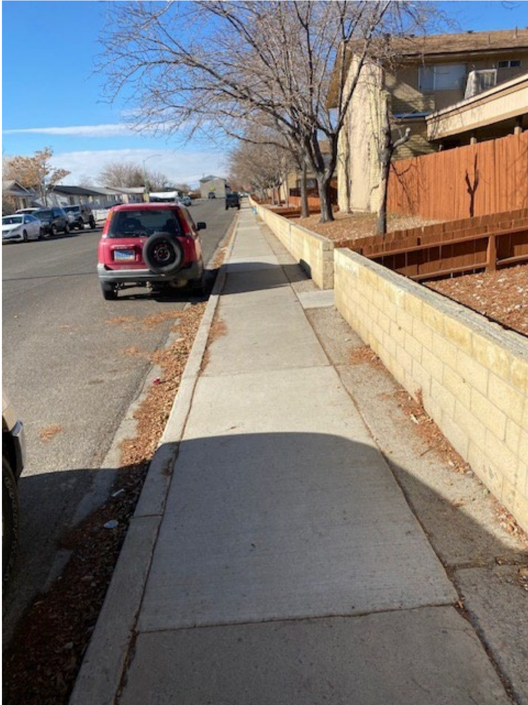
Repaired Sidewalk Sections
