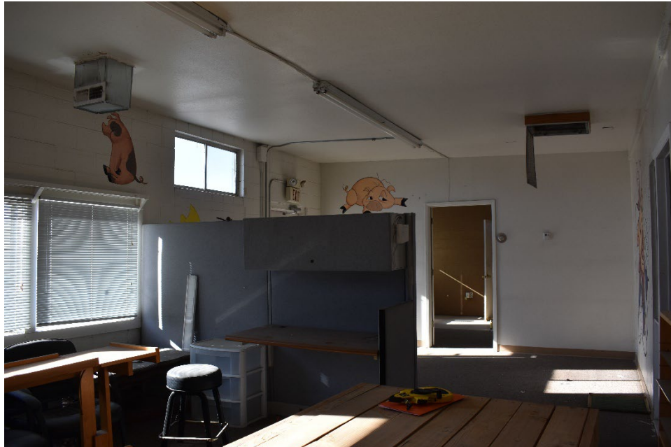
VIEW OF THE INTERIOR OF THE BUILDING
