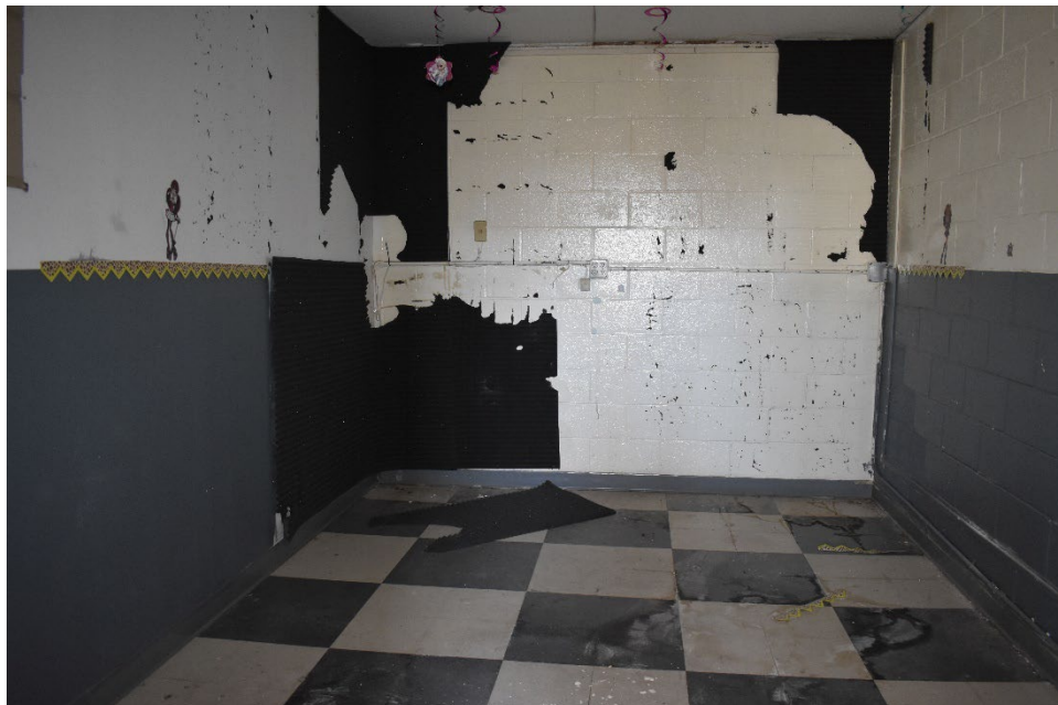
VIEW OF THE INTERIOR OF THE BUILDING
