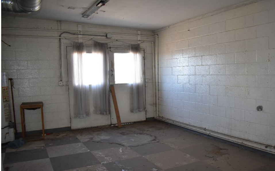
VIEW OF THE INTERIOR OF THE BUILDING
