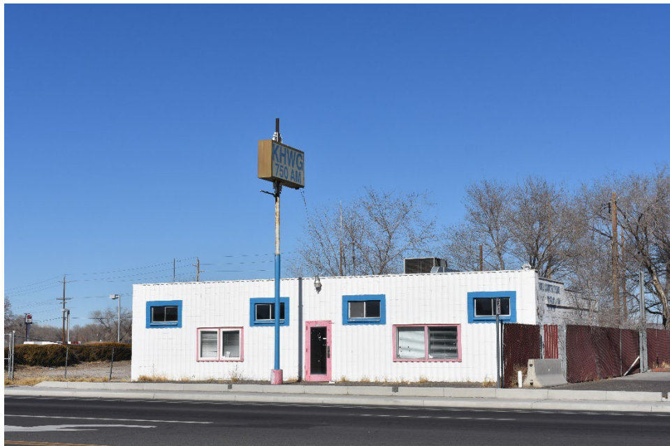
VIEW OF THE SUBJECT PROPERTY FACING NORTHWEST FROM WEST WILLIAMS AVENUE
