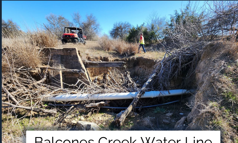
Balcones Creek Water Line Relocation
