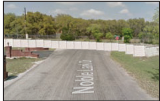
Figure 23 – Extended Existing Rock Fence
