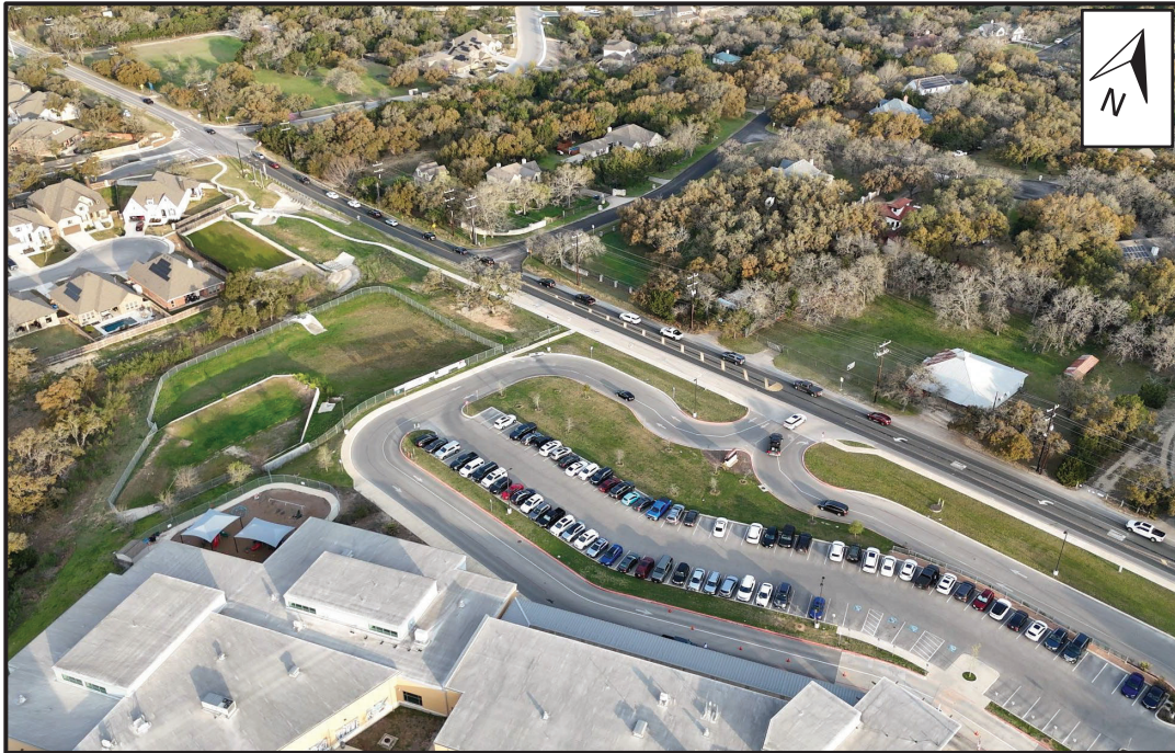
Figure 7 – Approximately 750 LF Queue at Dietz Elkhorn Rd and Square Gate (AM)
