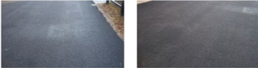
Pavement Condition 71 - 85 (Satisfactory)
