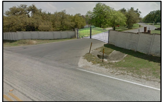
Figure 21 – Emergency Access Gate
