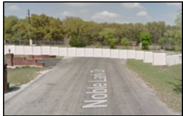
Figure 23 – Extended Existing Rock Fence
