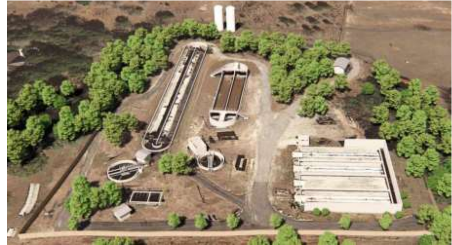
Aerial view of existing WWTP
