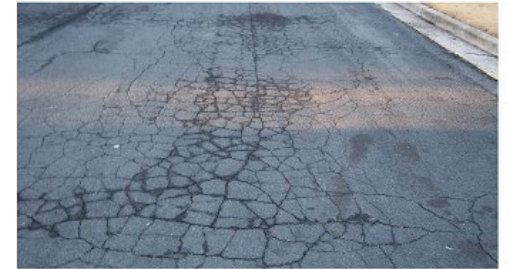
Pavement Condition 11 - 40 (Very Poor/Serious)
