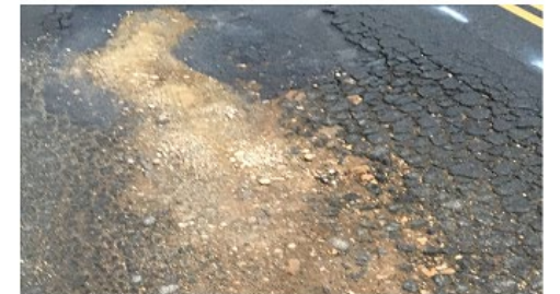
Pavement Condition 0 - 10 (Failed)
