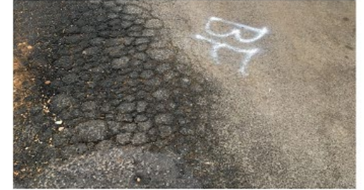
Pavement Condition 0 - 10 (Failed)
