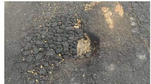
Pavement Condition 0 - 10 (Failed)
