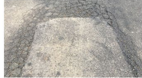
Pavement Condition 0 - 10 (Failed)
