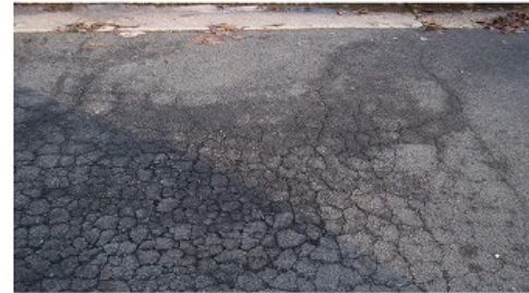
Pavement Condition 11 - 40 (Very Poor/Serious)
