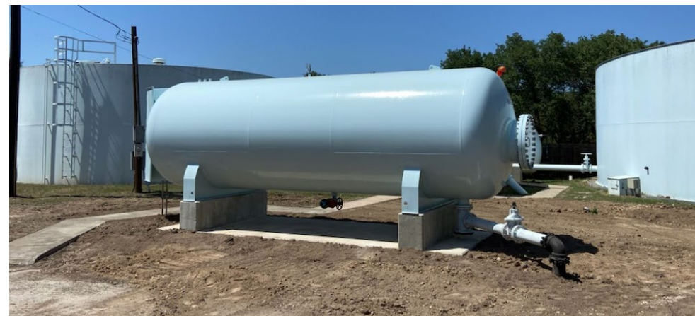
New 9000 gallon hydropneumatic tank at Plant #2
