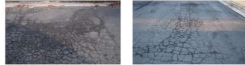
Pavement Condition 11 - 40 (Very Poor/Serious)
