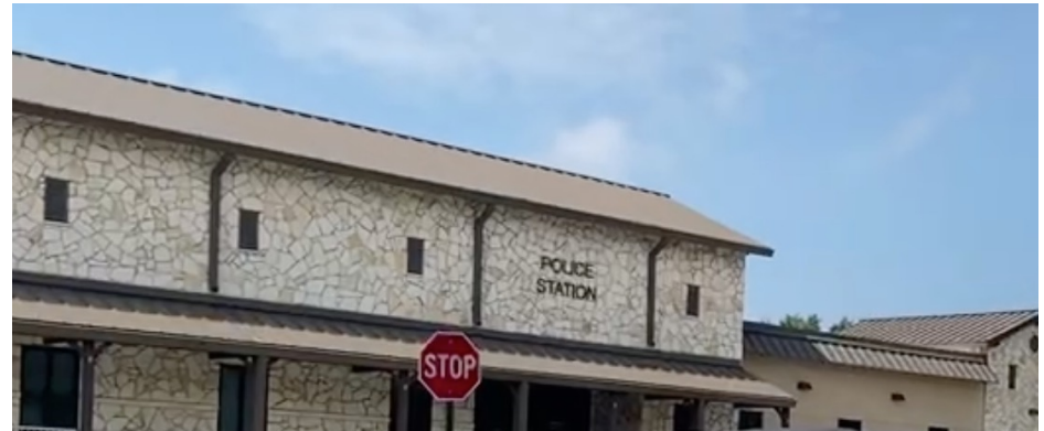
Existing Metal Roofs
