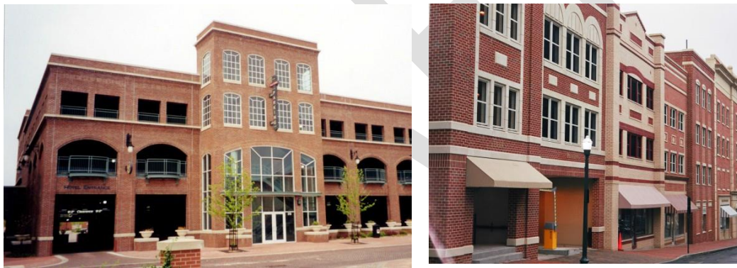
Figures 7-14-Images showing required Facade treatment of parking garages along Primary Frontages
