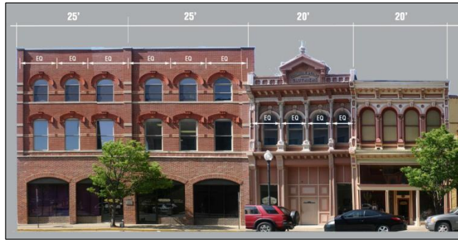
Figure 7-3 6.6 Illustration showing building articulation requirement
