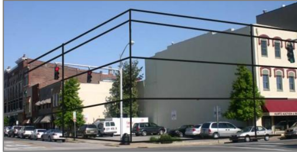
Figure 7-5-6.8 Figure showing how horizontal elements should match in the design of infill buildings.
