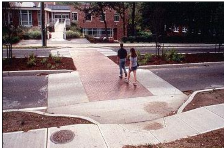
Picture 1: Raised Crosswalk speed reduction
