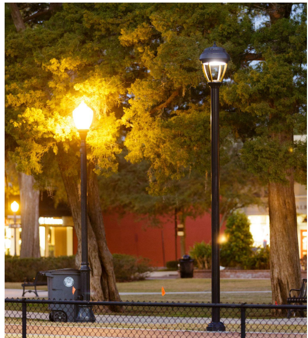
The photo depicts prohibited unshielded pedestrian walkway lighting versus fully-shielded lighting installed with 2700K CCT LED light.
