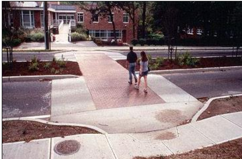
Picture 1: Raised Crosswalk speed reduction
