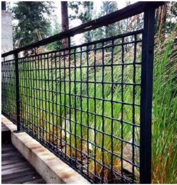
Steel & Wire Mesh Guardrail System
