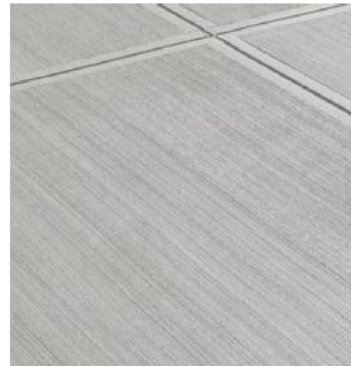
Concrete Flatwork broom finish
