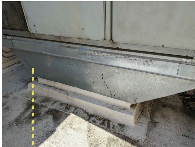
REPLACE UNIT AND ROOF CURB WITH APPROPRIATELY SIZED ROOF CURB
