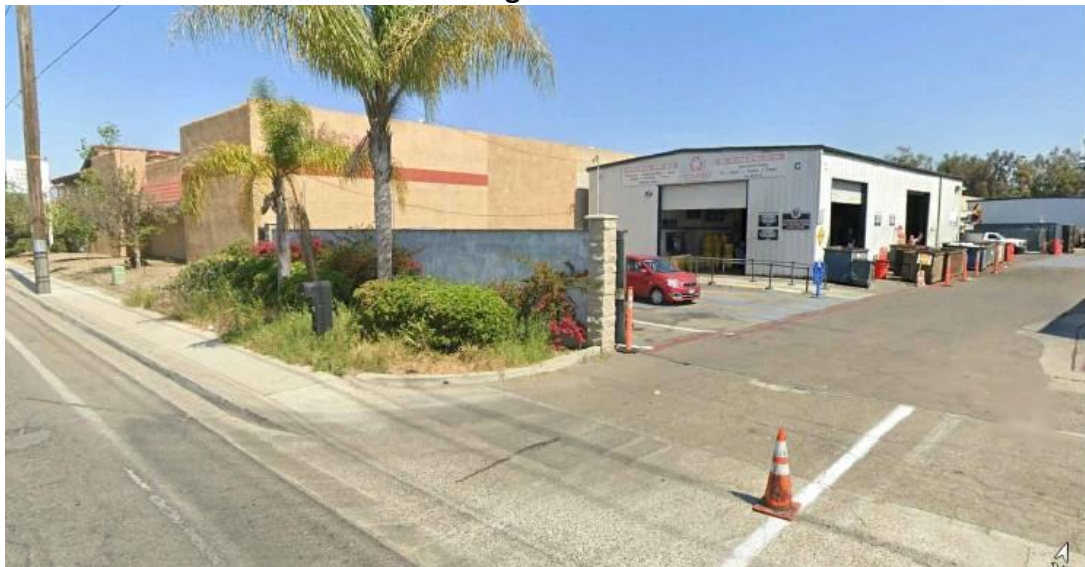
Looking northwest from W. Mission Road at existing CRV center
