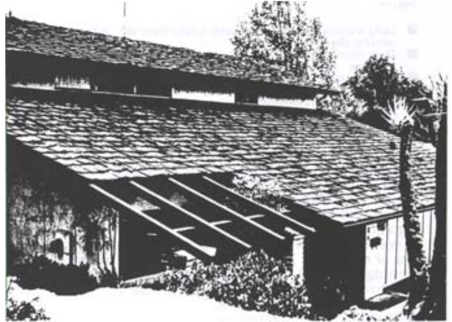
Good example of a shake roof.
