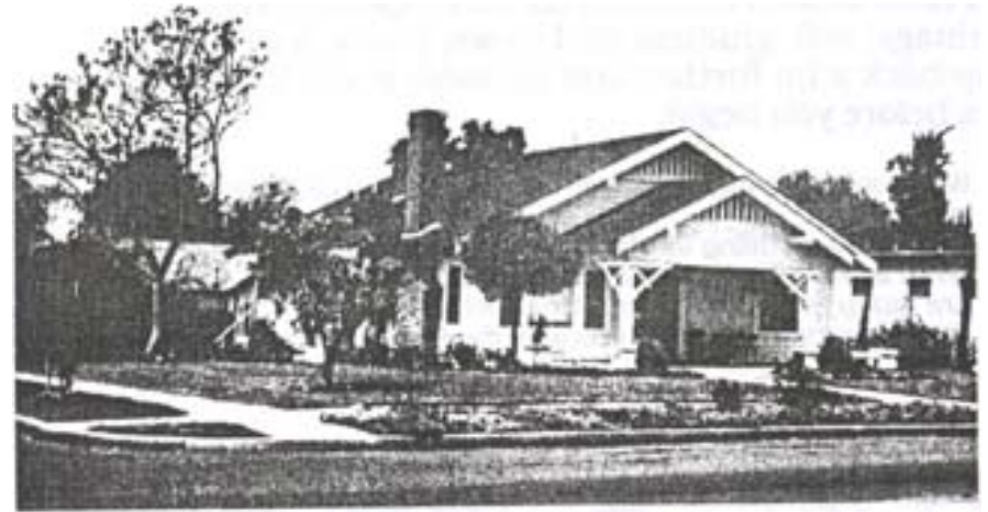
Traditional landscape pattern compliments the historic structure.
