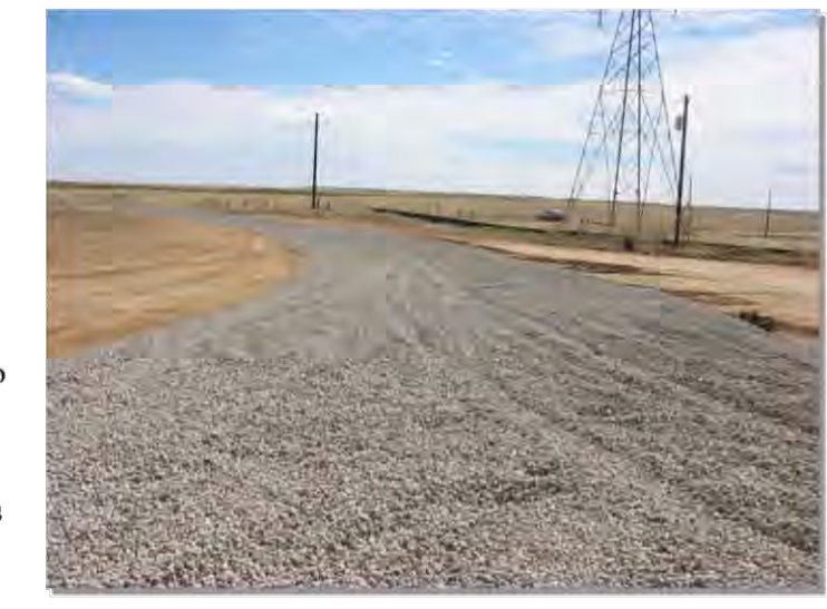
Photograph SCR-1. Stabilized construction roadway.
