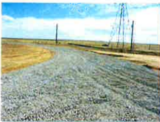
Photograph SCR-1. Stabilized construction roadway.
