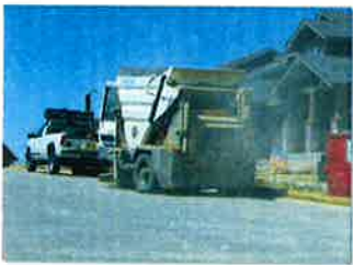
Photograph SS-1. A street sweeper removes sediment and potential pollutants along the curb line at a construction site. Photo courtesy of Tom Givens.
