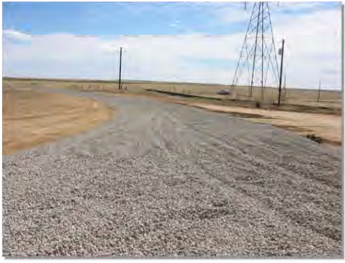
Photograph SCR-1. Stabilized construction roadway.
