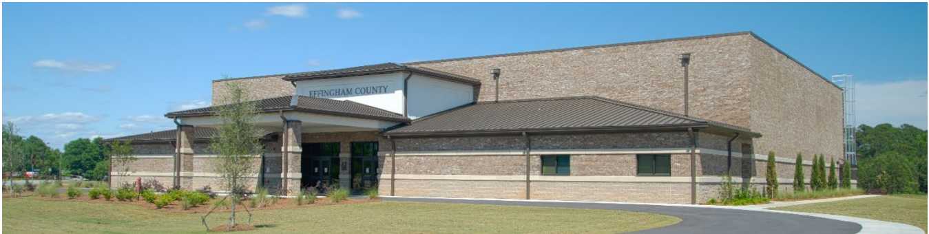
Effingham County Clarence E. Morgan Complex Phase 2 – New Gym, Springfield, GA
