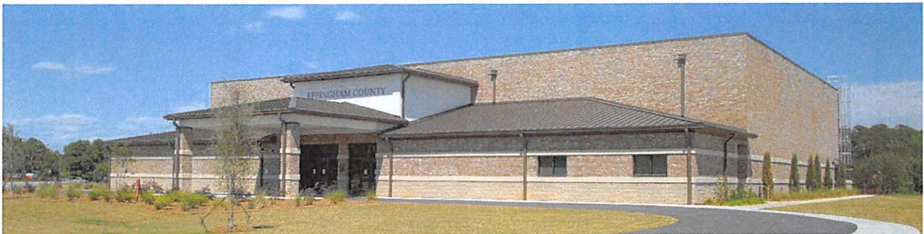
Effingham County Clarence E. Morgan Complex Phase 2 - New Gym, Springfield, GA
