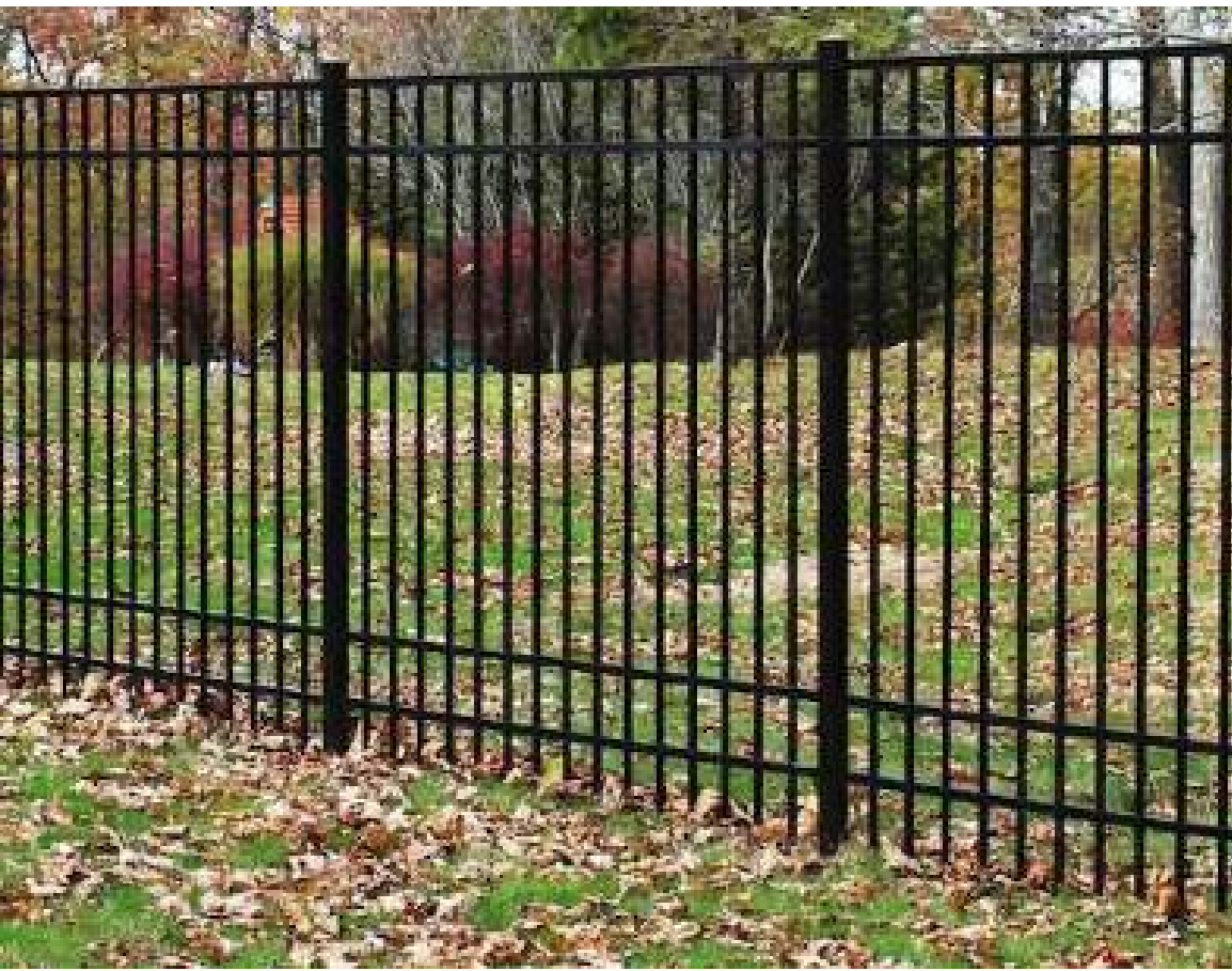
6' HT. VERTICAL PICKET SECURITY FENCING ALONG NATURAL AREAS AND OPEN SPACES
