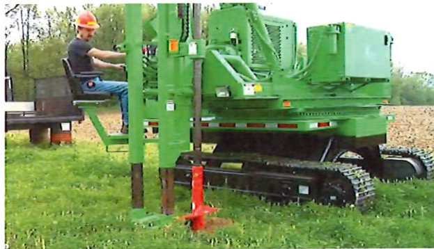
GRT Pile driver
