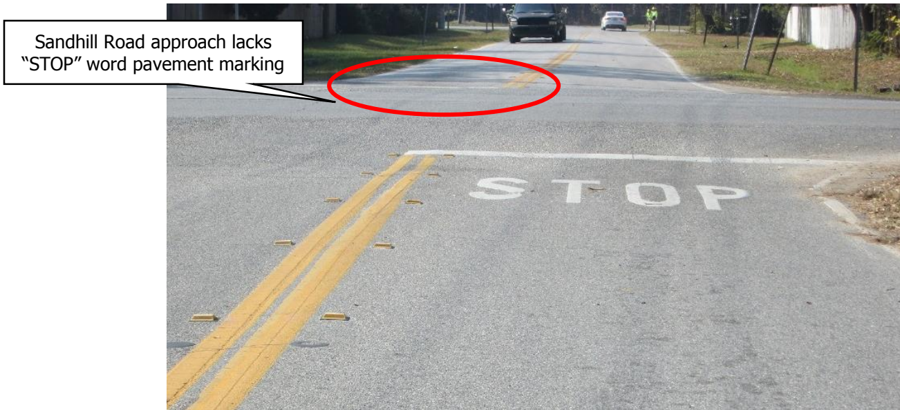
FIGURE 4-3. VIEW OF PAVEMENT MARKINGS AND RPMs ON MARLOW ROAD AT STUDY INTERSECTION
