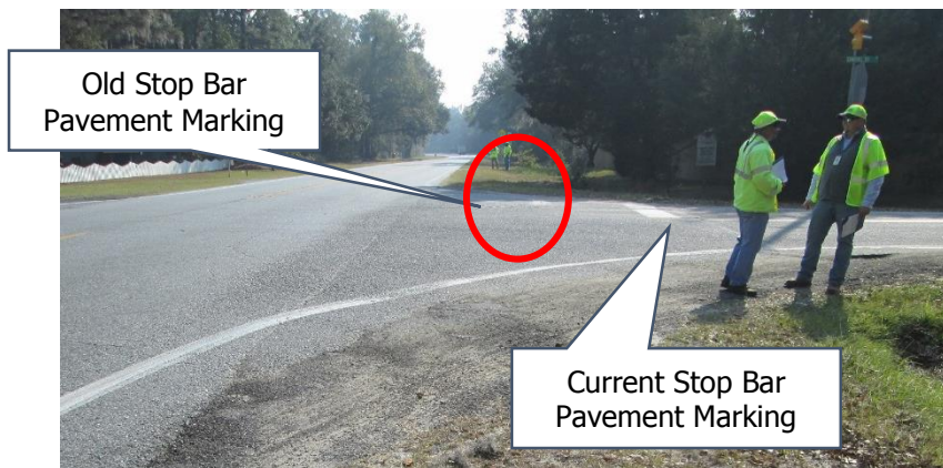
FIGURE 4-4. VIEW FROM SANDHILL RD. STOP BAR LOOKING SOUTHBOUND ALONG SR 17. NOTE THE VEGETATION, MULTIPLE STOP BARS, AND WHITE FENCE IN THE SOUTHEAST QUADRANT.
