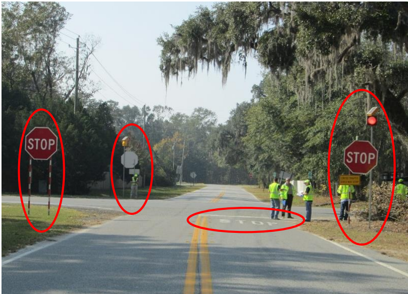
FIGURE 4-1. VIEW LOOKING ALONG WESTBOUND MARLOW RD TOWARD INTERSECTION WITH SR 17. NOTE THE RECENTLY INSTALLED OVERSIZED STOP SIGNS, SUPPLEMENTAL FLASHING BEACONS, AND PAVEMENT MARKINGS
