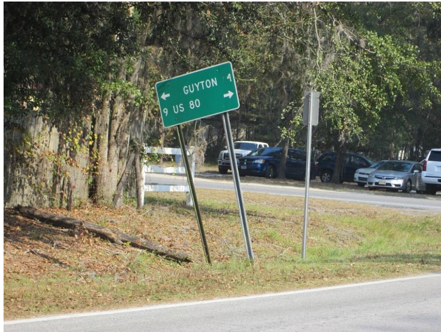
FIGURE 4-8. DAMAGED DIRECTIONAL SIGN ON NORTH SIDE OF SANDHILL ROAD APPROACH (NORTHWEST QUADRANT OF STUDY INTERSECTION)
