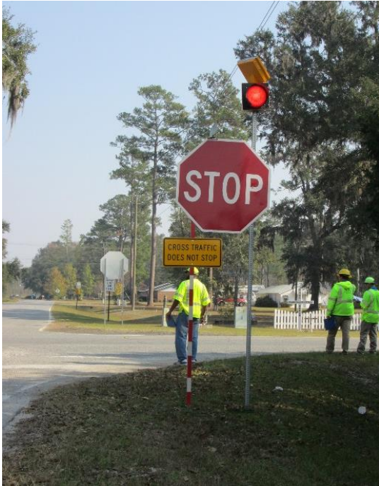
FIGURE 4-10. STOP SIGN ON SANDHILL RD WITH SUPPLEMENTAL "CROSS TRAFFIC DOES NOT STOP" SIGN AND FLASHING RED BEACON. NOTE THE REFLECTIVE RED AND WHITE STRIP. TO MEET CURRENT STANDARDS, A RED ONLY STRIP SHOULD BE ON BOTH POSTS.
