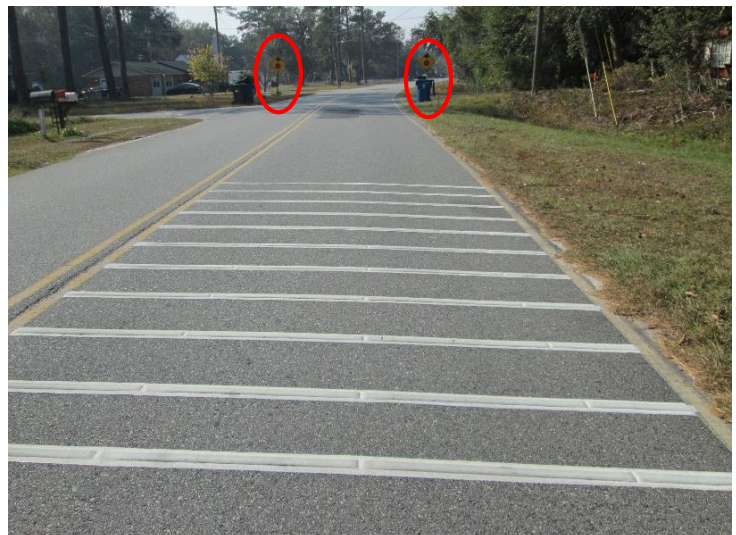
FIGURE 4-2. RAISED REFLECTIVE RUMBLE STRIPS ON MARLOW RD WITH ADVANCE WARNING "STOP AHEAD" SIGNS
