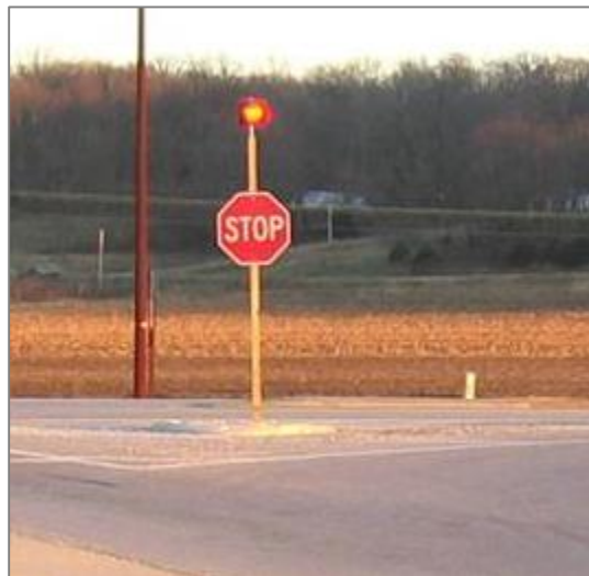
FIGURE 4-15. EXAMPLE OF A FLASHING BEACON MOUNTED ON A "STOP" SIGN. SOURCE: FHWA PUBLICATION HRT-08-044 3
