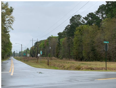
Georgia Power corridor following Central Avenue out of Guyton.
