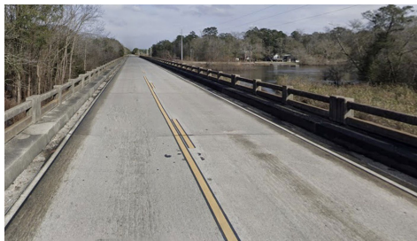
Existing conditions of GA-119 bridge over the Ogeechee River near Guyton.
