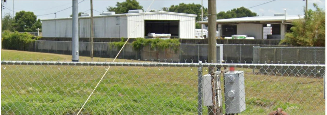
Exhibit 8 – Existing Fence Along North Property Line
