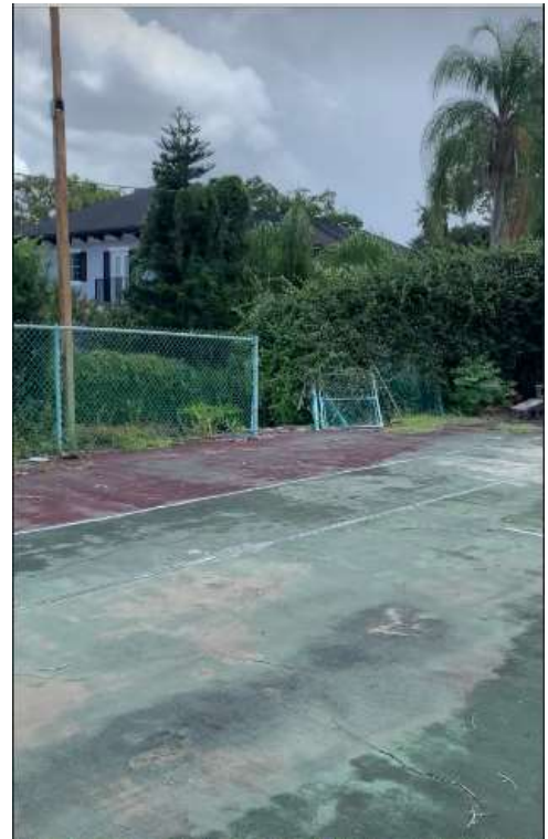
Looking at Southeast corner of court
