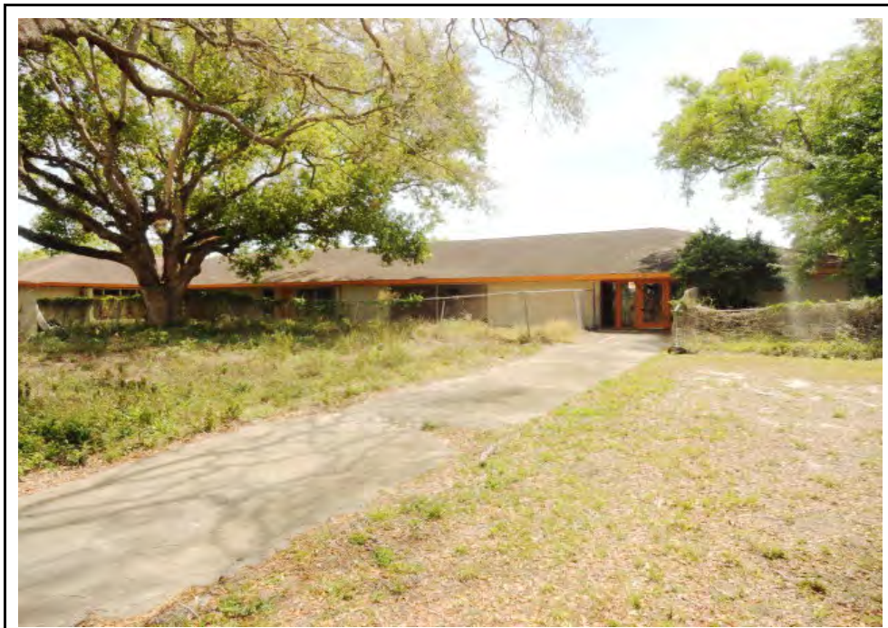
Secondary Access on Lemon St
