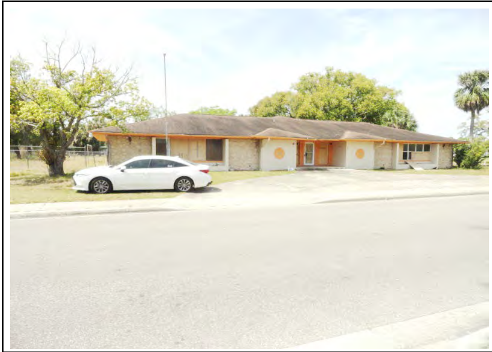
Main Entrance on S West St
