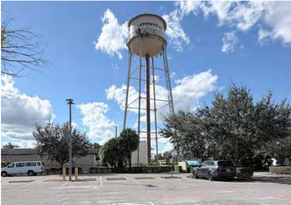
Eatonville Water Tower (Built 1956)
