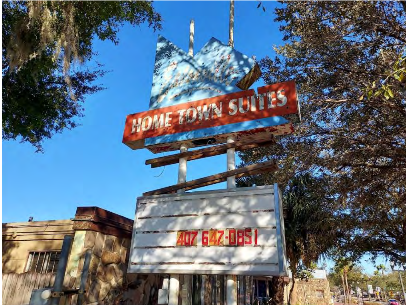
Smith's Eatonville Motel was built in 1967 and is a potential Mid-Century Modern National Register eligible resource.
