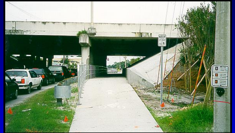
Pedestrian Access Under I-4
