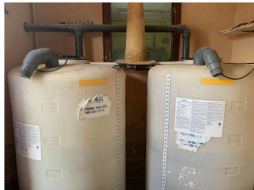
Photo 4-3: Chlorine Chemical Feed System
