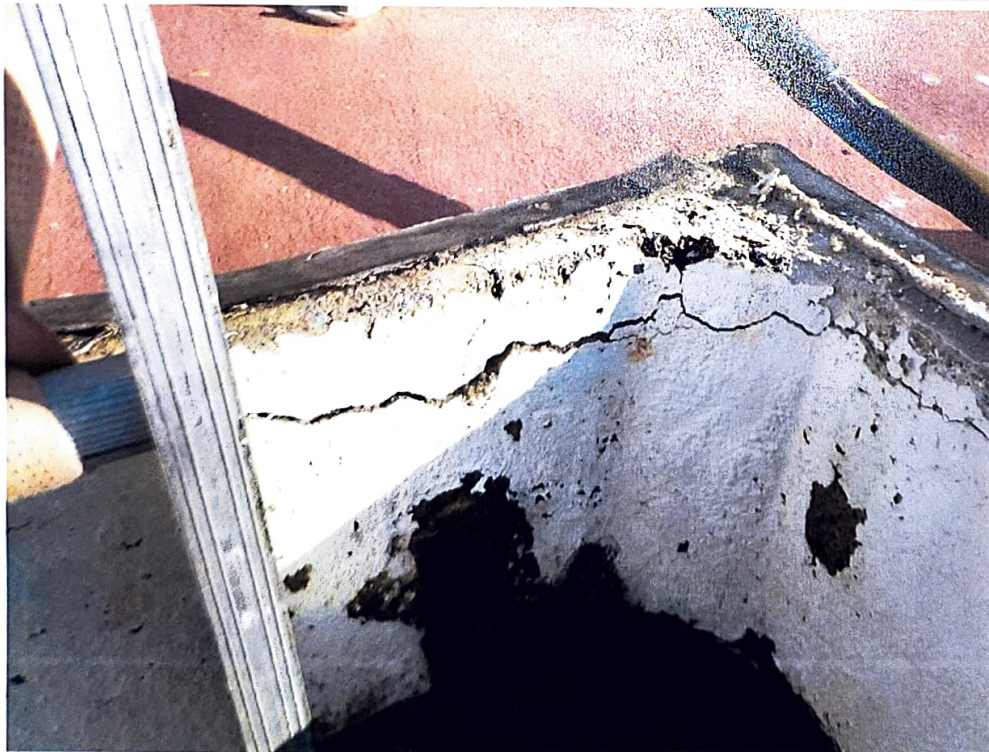
Primary Access Hatch (note cracking)
