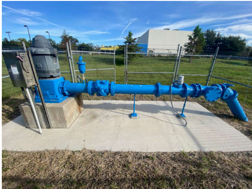
Photo 4-1: Wellhead Discharge Assembly
