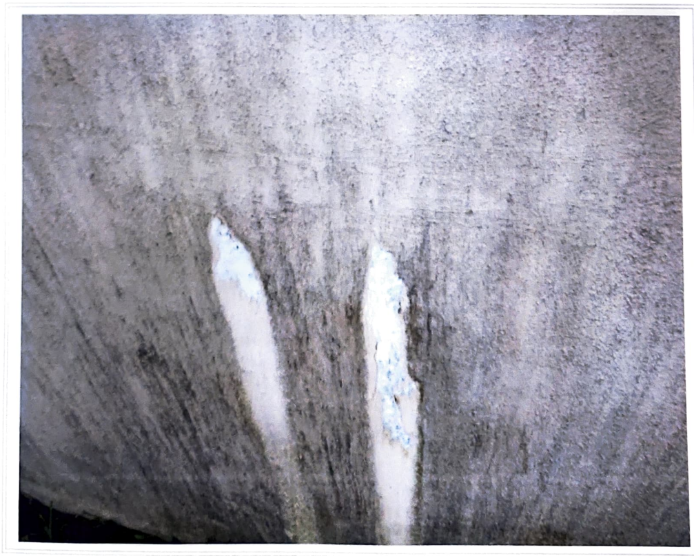
Staining and Cracking with Efflorescence on Exterior Wall
