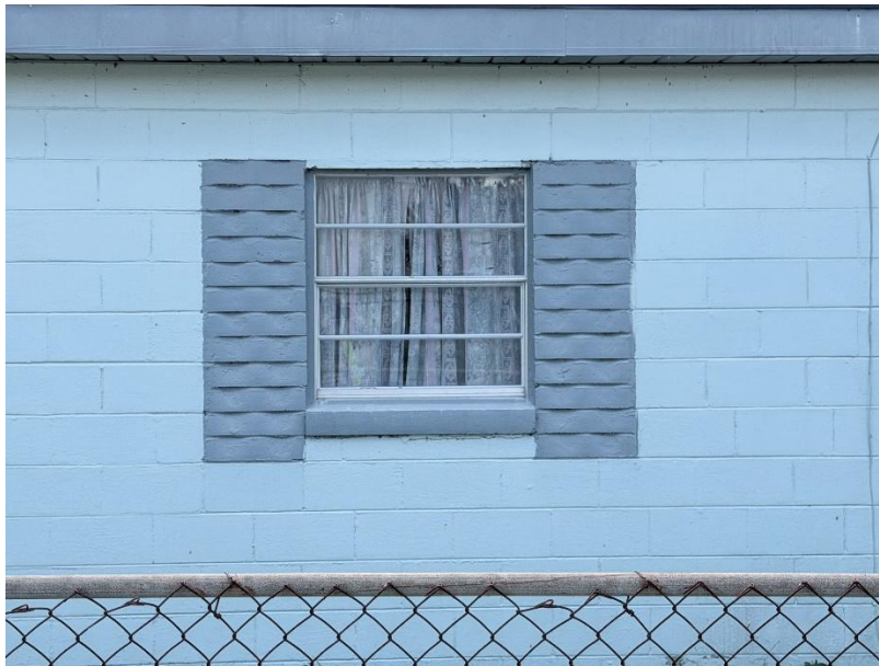
Figure 50. 10 Moseley Avenue with embedded shutters. | Planning 2 Preserve
