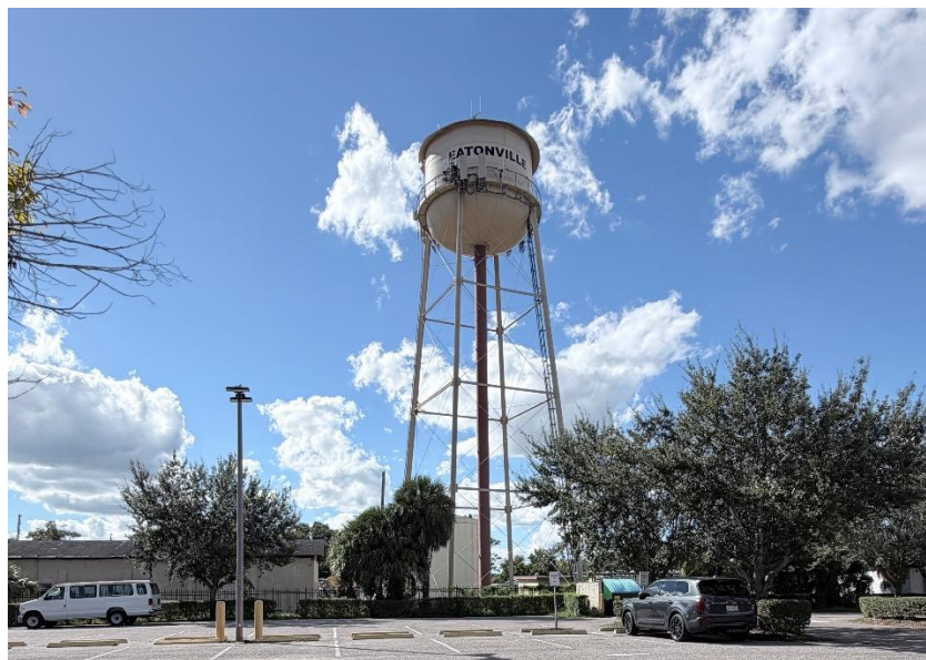
Figure 55. Eatonville Water Tower, 21 Moseley Avenue. | Planning 2 Preserve
