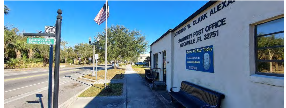
Eatonville Community Post Office
