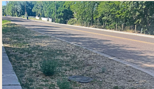
Town of Eagar – Main Street Sewer
