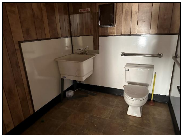
Restroom (Building B)
