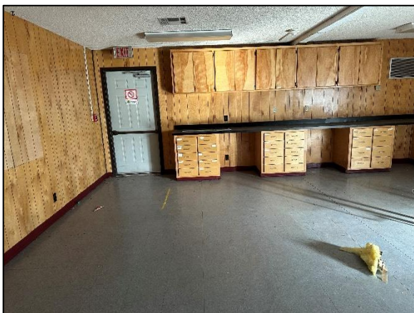
Interior View (Building C)
