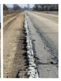
In spite of this, the foundation of the roadway appears to be in fairly good condition. The ride is rough in places, primarily due to the degradation of the surface course – not due to foundation failure (see photos, below). It appears that little, if any foundation work would need to be performed. A surface treatment of the appropriate application could easily bring this facility back to a serviceable condition.
