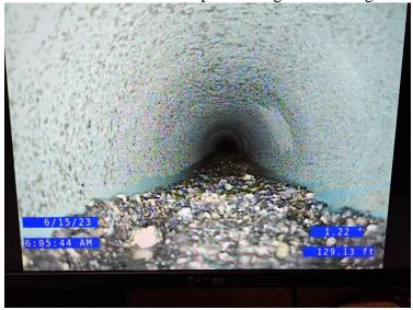
This is an example of a pipe we had found earlier this year that the soil and gravel that had leaked into a sewer pipe though a hole found in our manhole. Popping the lid on the manhole you wouldn't have been able to catch it cause is was backing up down stream of the sewer main.
