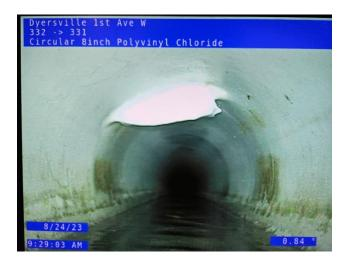
We found that our sewer main on 1<sup>st</sup> Ave W had been hit by a directional drilling company. This is inspecting down the line and found this bulge in the top of the main.
