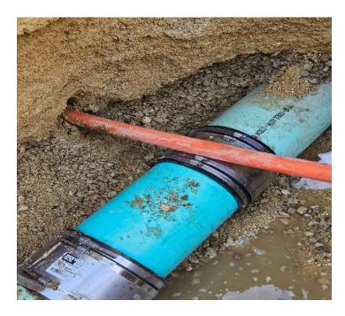
By Finding this and check locate tickets we were able to find out who hit it and then we had Krapfls come in and dig it up and make the proper repairs before more damage was done. With a hole like that we could have a massive back up with that being a main sewer run and could have caused the road to undermine and collapse causing more damage and possible injury.
