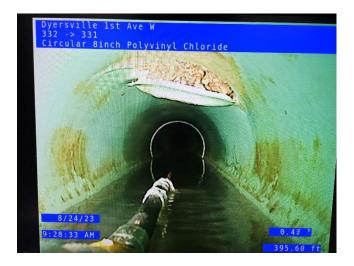
This is looking out the rear of the camera showing the crack with exposed soil and gravel. The cable you see in the pipe is the cord for the camera.
