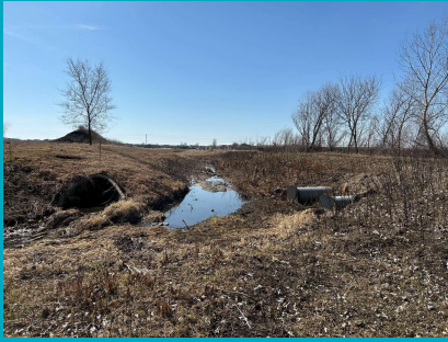
Existing Outfall looking south
