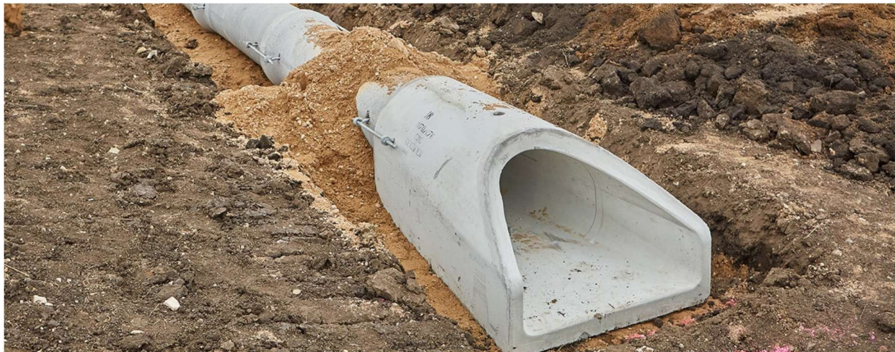
Figure 7: Concrete pipe with apron
