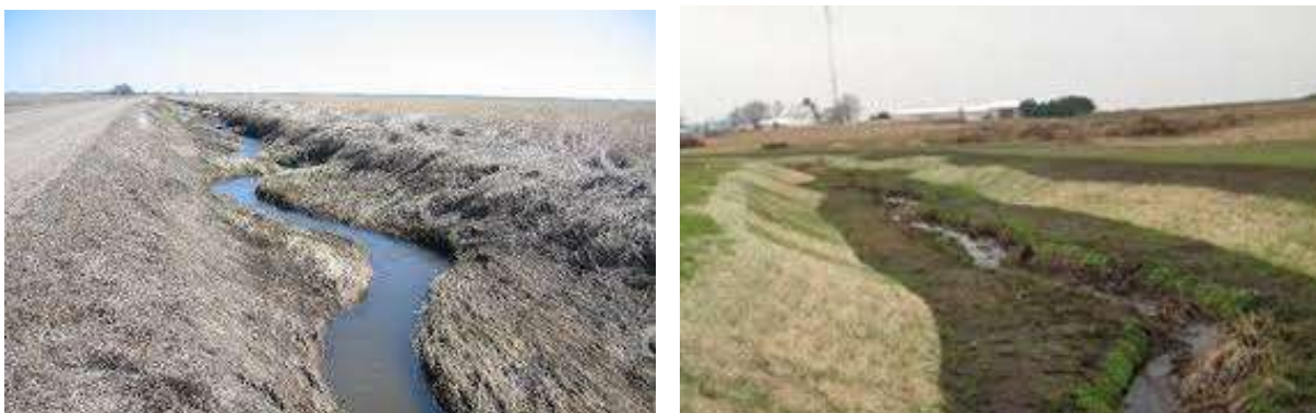
Figure 4: Examples of Two-Stage Ditches with Meandered Main Channel
