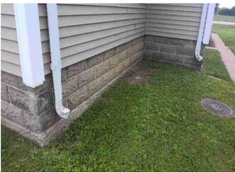
The gutters on the composition shingle roof should be cleaned and serviced to drain properly. I would suggest some type of gutter guards to keep materials out of the downspouts to promote positive drainage.
