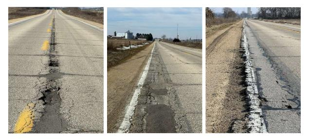
In spite of this, the foundation of the roadway appears to be in fairly good condition. The ride is rough in places, primarily due to the degradation of the surface course – not due to foundation failure (see photos, below). It appears that little, if any foundation work would need to be performed. A surface treatment of the appropriate application could easily bring this facility back to a serviceable condition.
