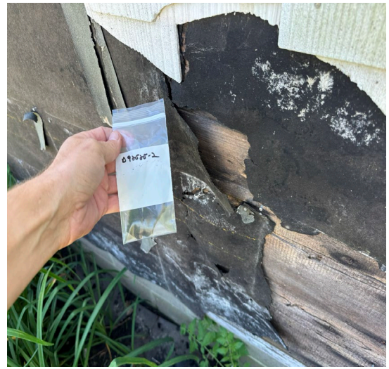
Sample D92525-2: Exterior tar paper behind siding negative for asbestos.
