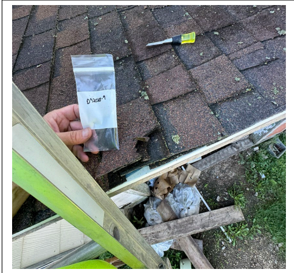
Sample D92525-9: Singles/ice dam on roof negative for asbestos.
