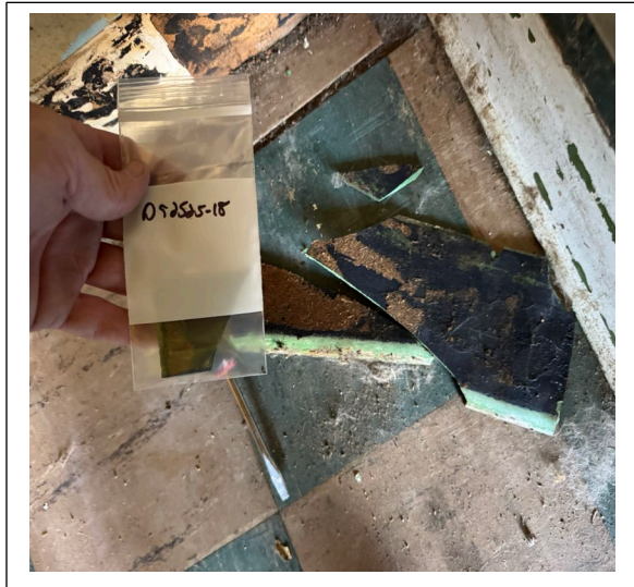
Sample D92525-18: Vinyl base/adhesive in main room negative for asbestos.
