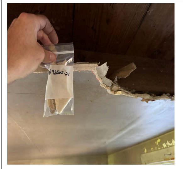
Sample D92525-21: Plaster/drywall backer in kitchen ceiling negative for asbestos.
