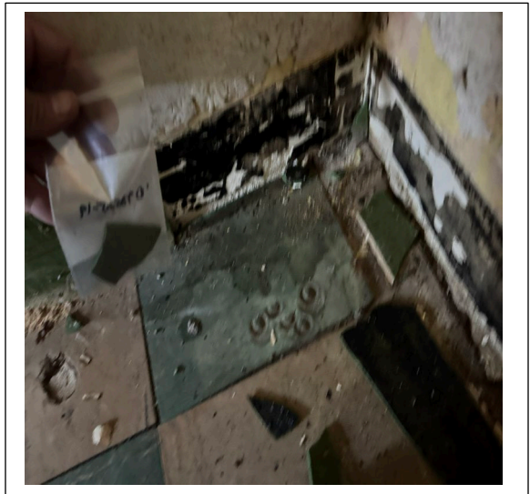
Sample D92525-19: Base cove/adhesive in kitchen negative for asbestos.
