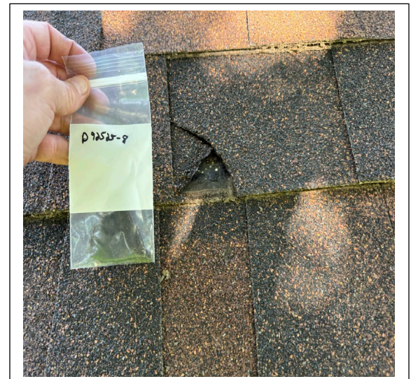
Sample D92525-8: Singles/ice dam on roof negative for asbestos.
