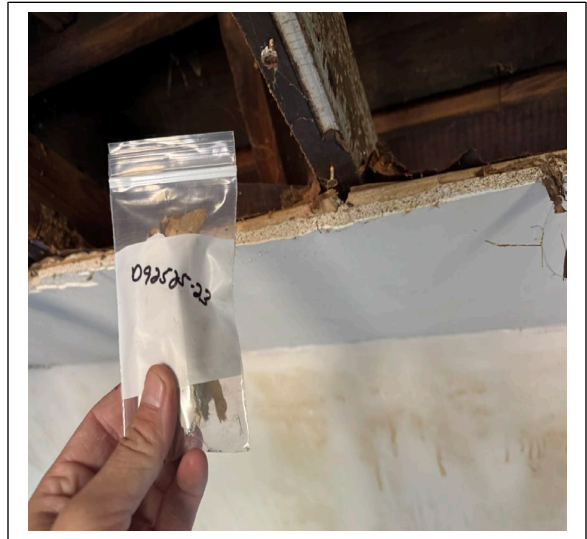
Sample D92525-22: Plaster/drywall backer basement landing <1% asbestos (PC).
