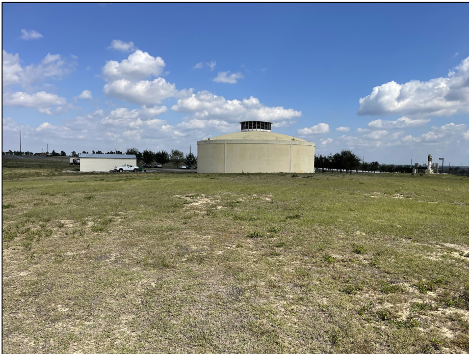
Figure C-2. Hickory Walk WTP Ground Storage Tank
