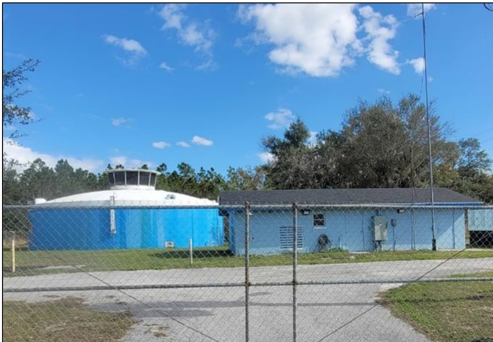
Figure C-4. Riner WTP Ground Storage Tank and HSPS Building
